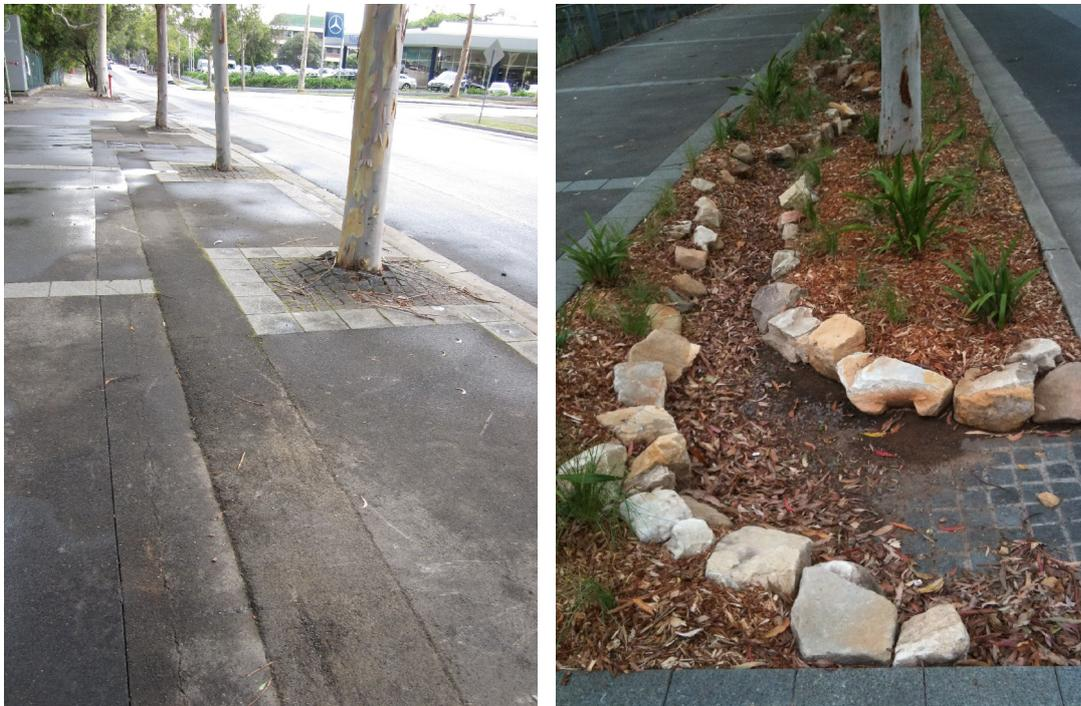
**Figure 1: Before and after installation of the first raingarden**
