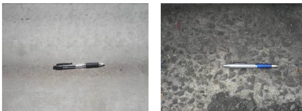
Figure 1. Photo of the concrete surfaces at St Columbans Green constructed in 2008 (left) and Currong Place constructed in 1981 (right).
