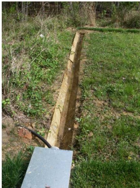
Figure 1. Level Spreader-VFS (a), Recollection Trough, and Weir Box(b).
