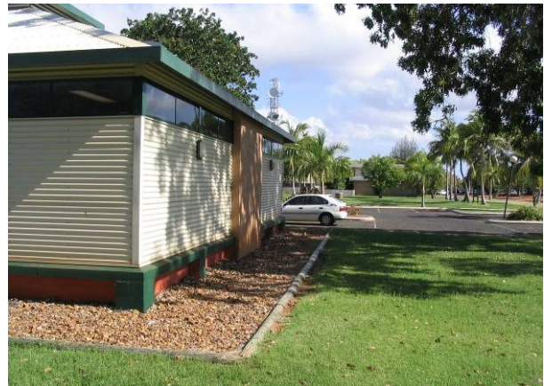
Figure 7. Pervious surface underneath a gutterless roof, Shire of Broome offices, Broome. (Photograph: Allan Ralph, Shire of Broome 2005.)
