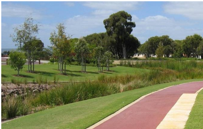
Figure 4. Vegetated swale in Gosnells, making use of native species in a parkland setting. (Photograph: Department of Water 2004.)
